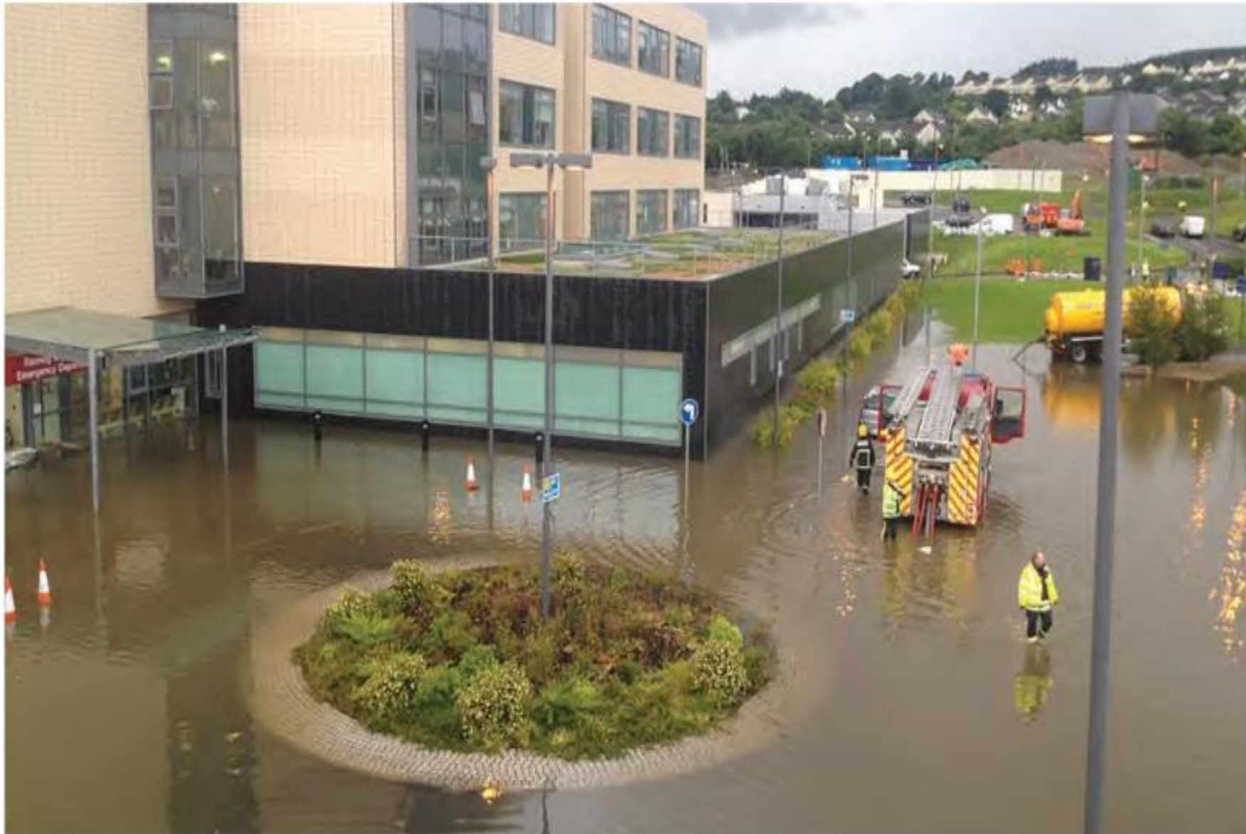
Figure 8.4 Letterkenny hospital after floods in 2013, when 40% of hospital services had to be taken out of clinical use. (Source: McGinley (2014), Photo Declan Doherty)
